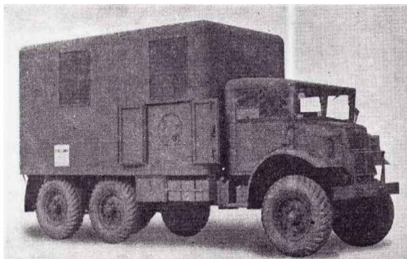
Afb 45. Lorry, 3-ton, 6-wheels, 160-in WB, Machinery "Z". (3-ton, 6x6, 160" W.B.)
